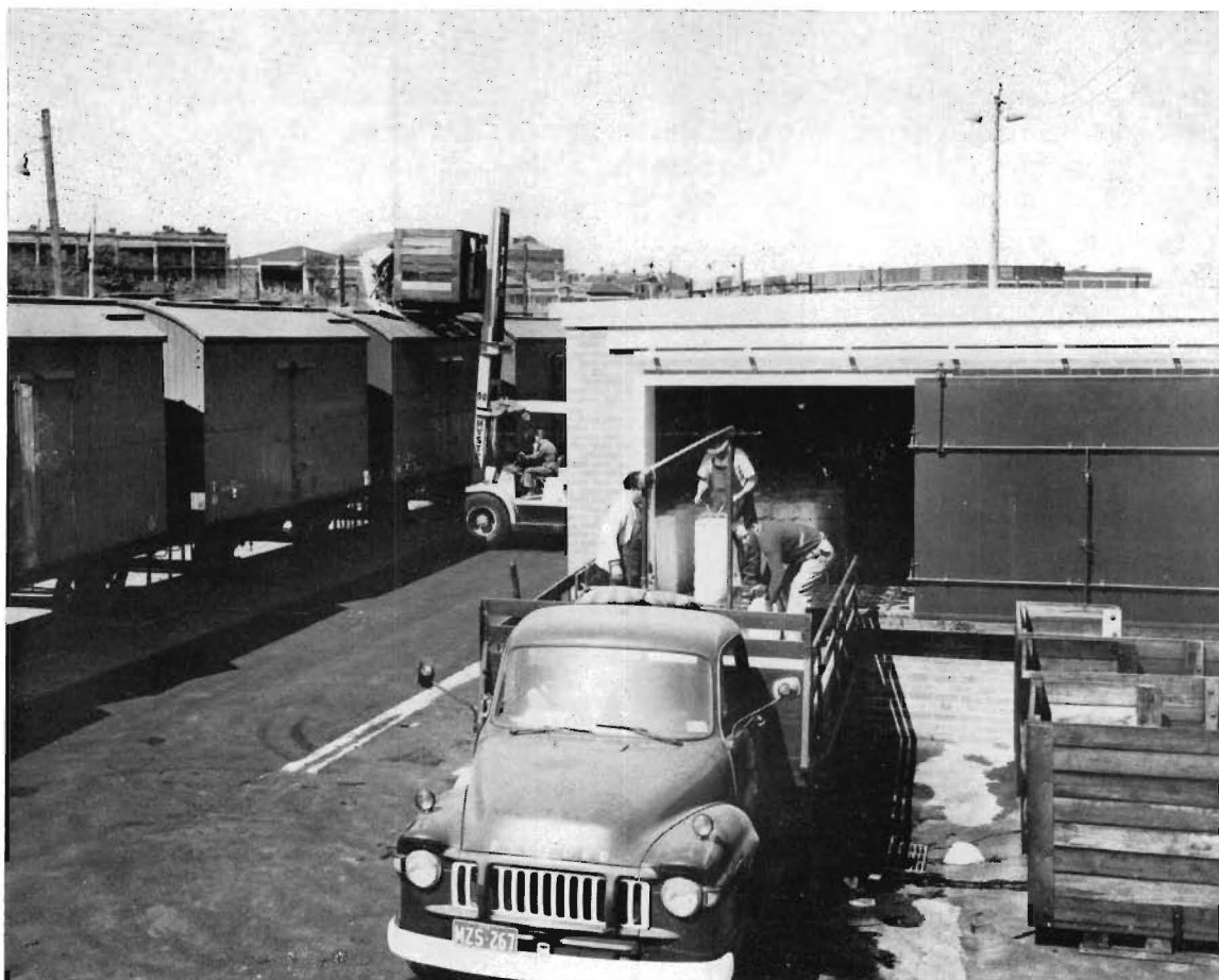
New facilities for icing refrigerator vans, Melbourne Yard.
