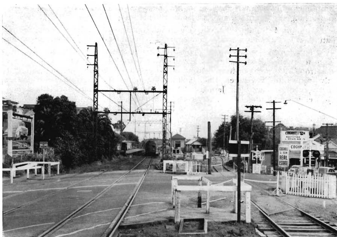
Commencement of grade separation project at Canterbury Road, Canterbury, with temporary track and platform on right.
