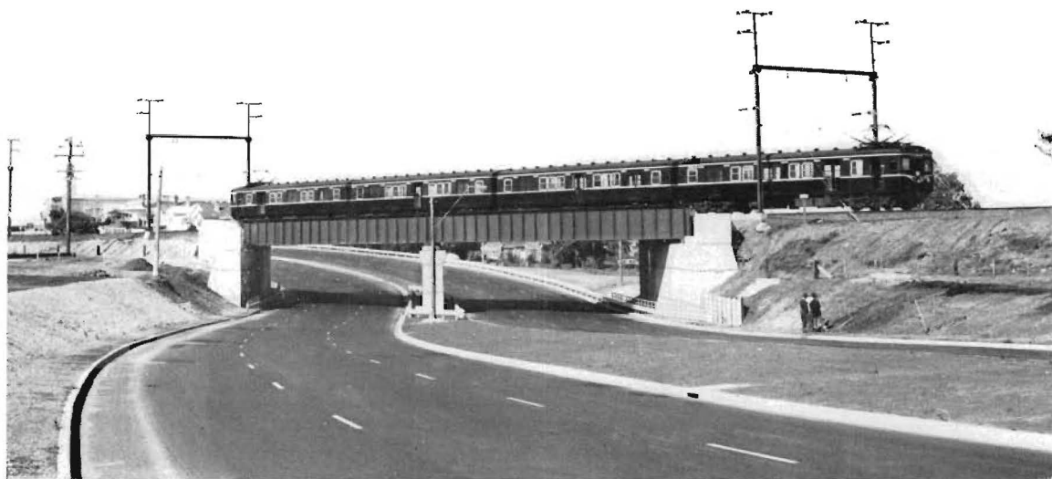
New bridge over Nepean Highway, Mordialloc.
